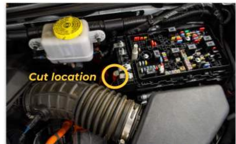
Positive supply cable with fuse box cover removed
