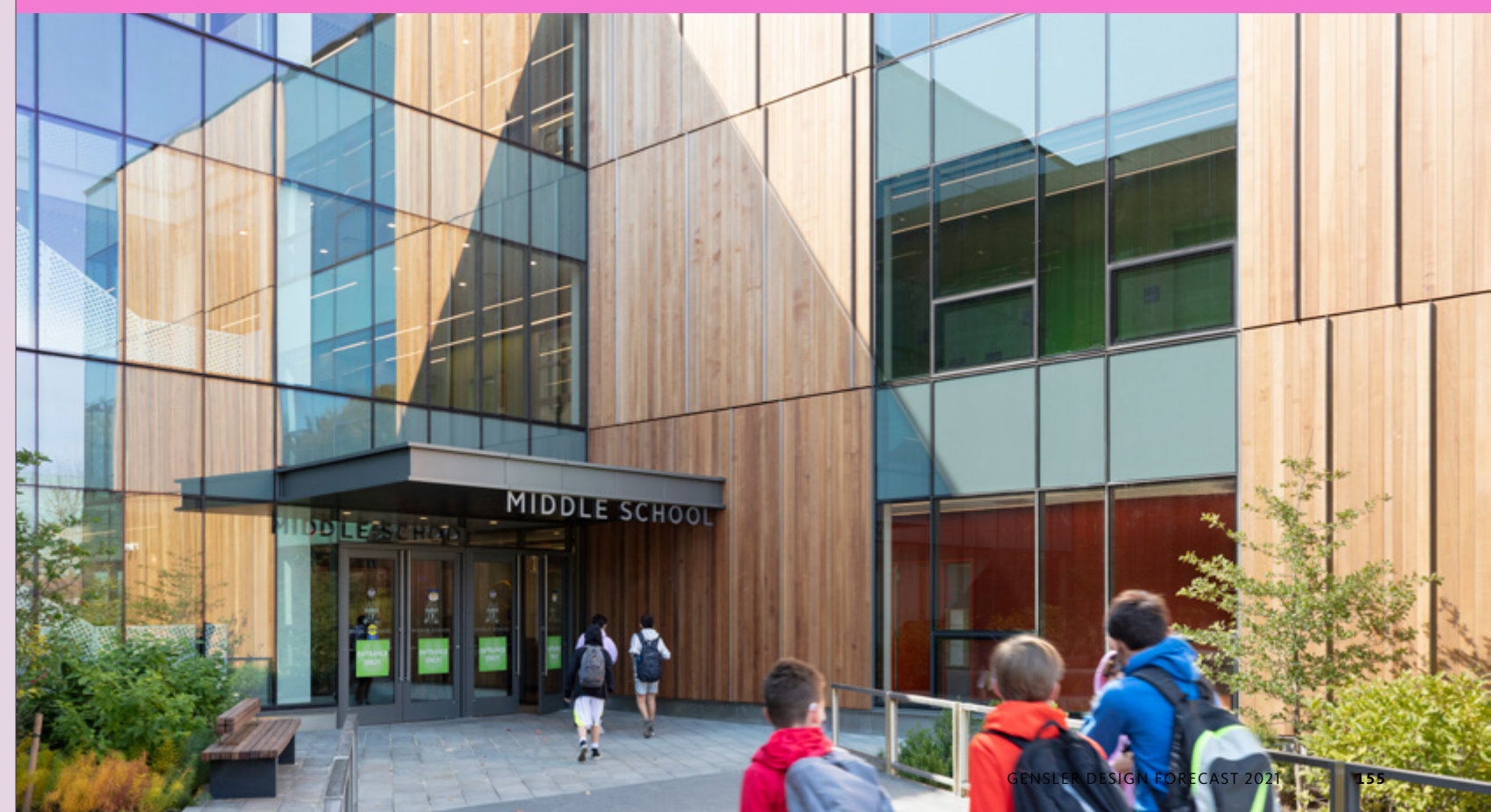
DWIGHT-ENGLEWOOD VILLAGE & MIDDLE SCHOOL, ENGLEWOOD, N.J.
