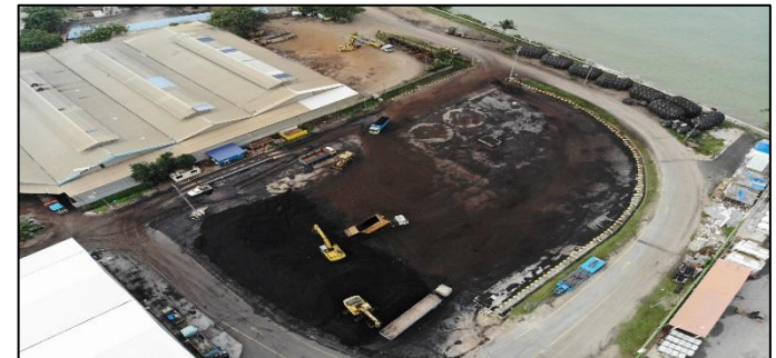
Interlocking Pavement and Kerb at Open Yard
