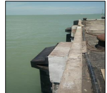
Replacement of New Fender and Improvement of Kerb jetty
