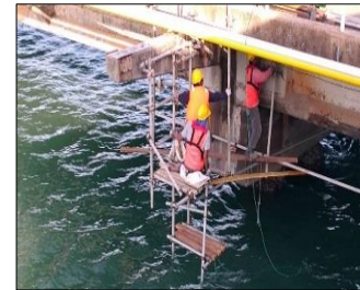
Installation of Framework
