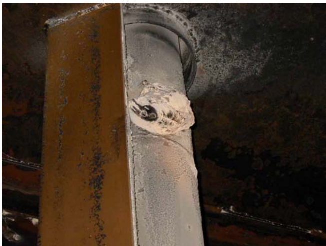
Figure 5: Sulfuric Acid Deposits together with ash have completely blocked SO 3 flow from injector nozzle
