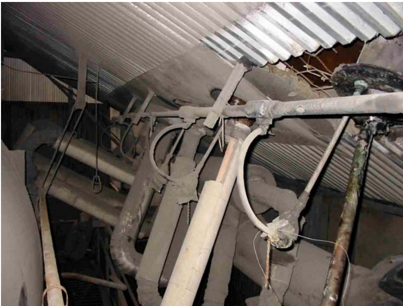
Figure 8: This shows insulation being completely removed from SO 3 piping leading to the injector. The sulfuric green acid on the exterior indicates failure of the SO 3 piping due to acid attack. This unit also shows a bottom of the duct installation. Further complicating matters.
