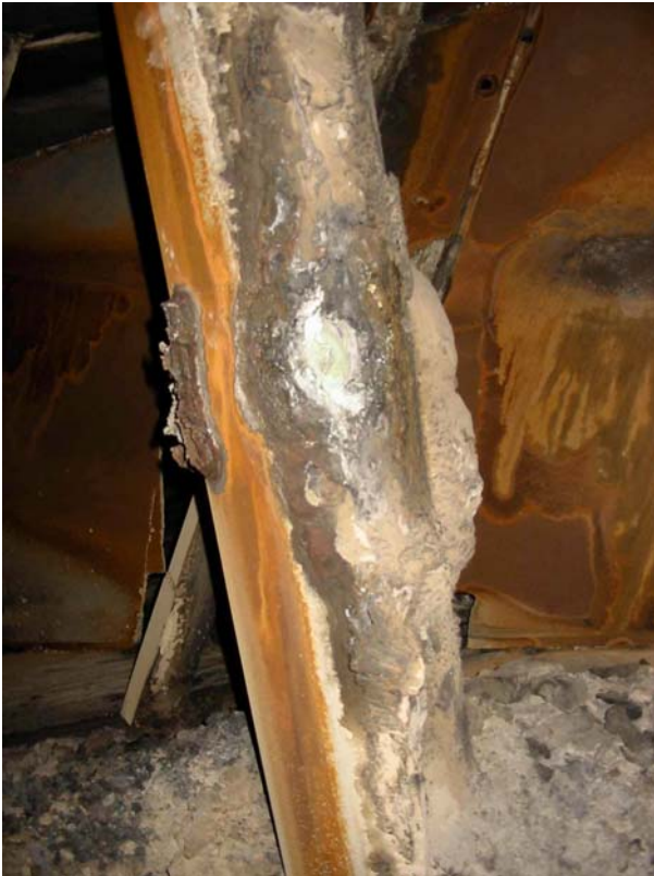
Figure 9: Injector inside of duct with insulation problems on the SO 3 line leading to injector
