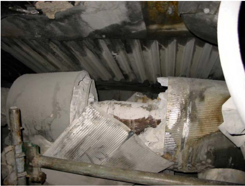
Figure 7: Damaged insulation on SO 3 piping leading to injectors
